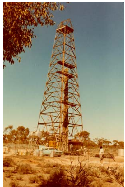
LY 44 under Lee C Moore K Frame derrick near Kambalda 1967 – 60 ft pull
