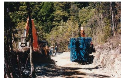
Finally the rig arrived at site.
